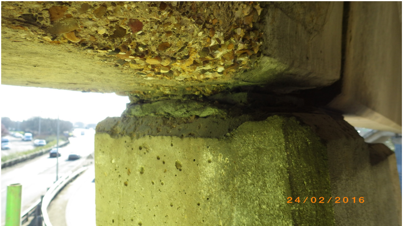
Figure four: Sheets of poor concrete have spalled from the piers exposing the corroded reinforcement
