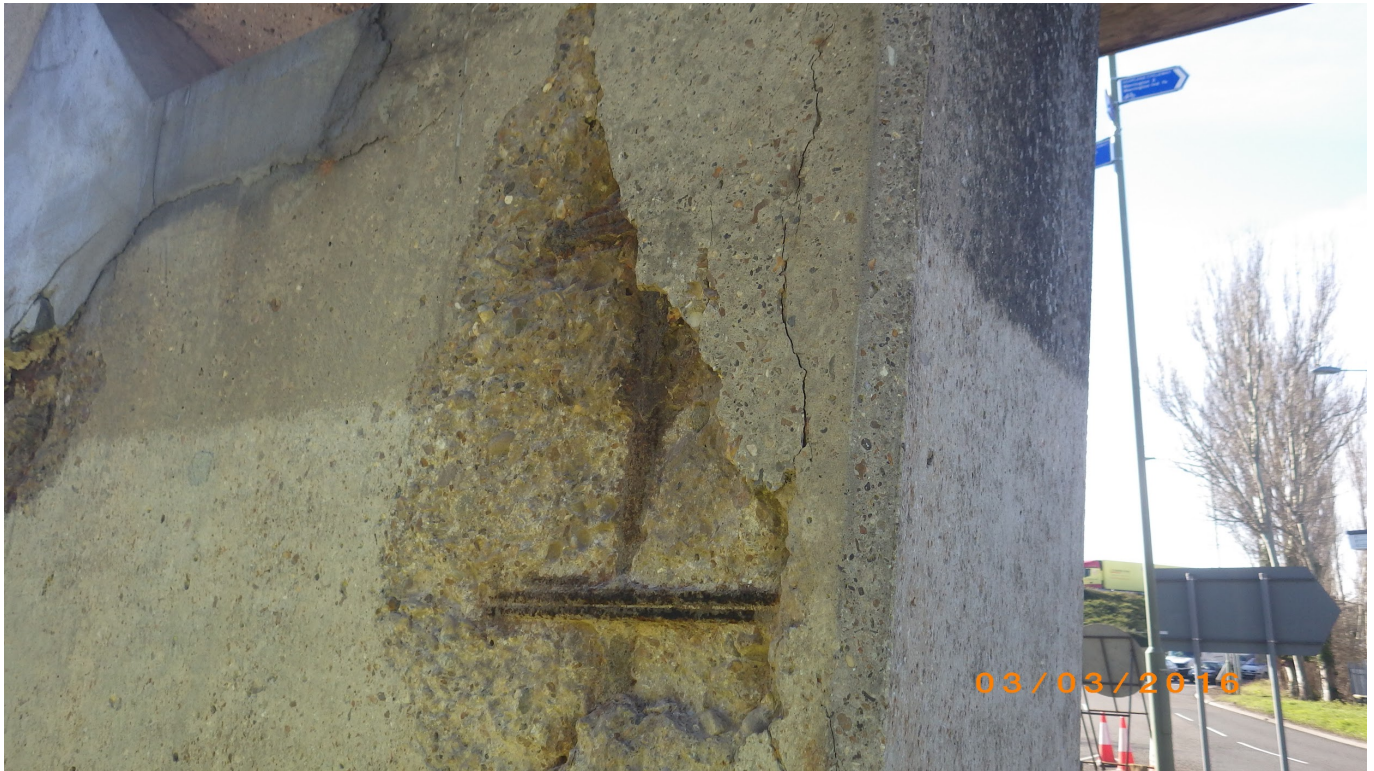
Figure six: Very significant cracking to already repaired areas of the fork of the piers where stresses are at their maximum.
