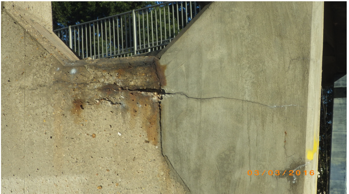
Figure six: Very significant cracking to already repaired areas of the fork of the piers where stresses are at their maximum.
