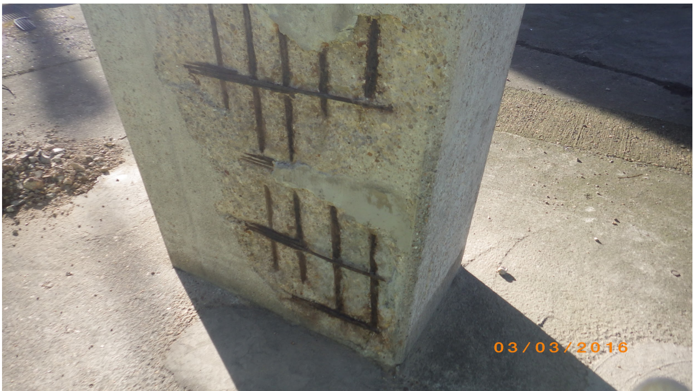
Figure four: Sheets of poor concrete have spalled from the piers exposing the corroded reinforcement
